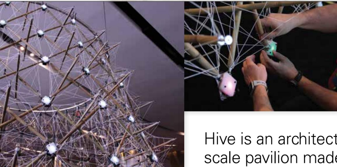
Hive is an architectural-scale pavilion made from 224 tensegrity parts built by humans and robots working in close collaboration.
